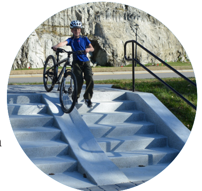
Bike runnels are smooth u-shaped guideways adjacent to a staircase that allows cyclists to roll their bikes as opposed to having to lift and carry them.
